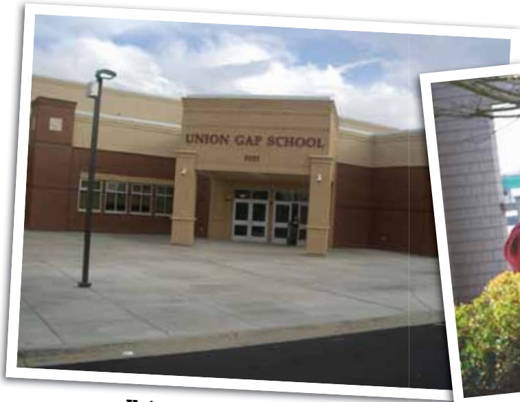
Union Gap Elementary
